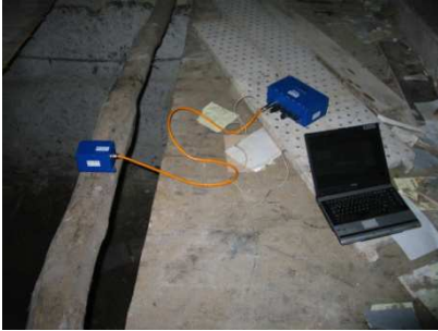
Fig. 1. Frequency measurement on a single timber beam.
