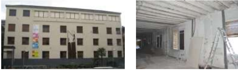
Fig. 1 Exterior building front view and beams of the second floor
