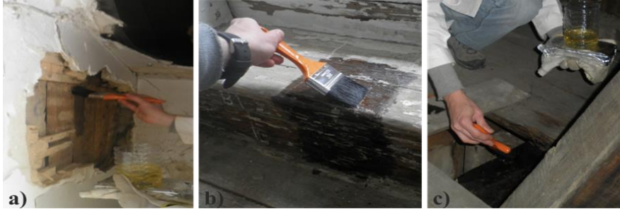
Fig. 1. Application of consolidant a) Wall; b) Staircase; c) Pavement beam 1 [18]
