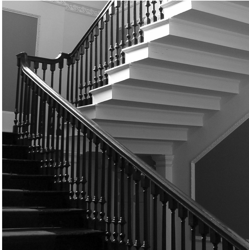
Figure 2 Cantilever stair at Lytham Hall, by John Carr, 1758.
