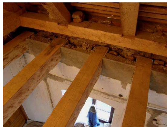
Fig. 16 Detail of the aired space around beam heads
