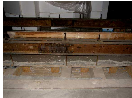
Fig. 3 Steel girders holding the ceiling after the reconstruction in the 1970s
