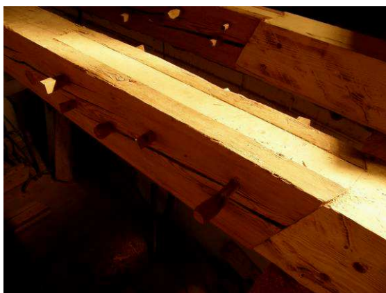
Fig. 13 Detail of all-wood joint after joining
