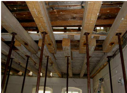
Fig. 2 Parts of ceiling beams inserted during the reconstruction in the 1970s
