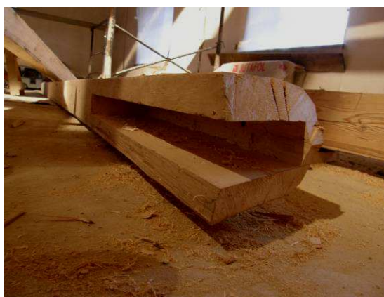
Fig. 14 Detail of hand-made mortise
