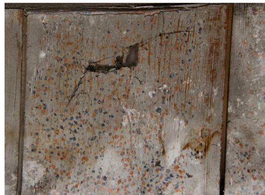
Fig. 5 Detail of the colour decoration on limewash on the decking planks
