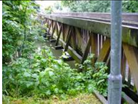
Fig. 5: Typical timber bridge to be inspected because of decay (although made by tropical hardwoods).
