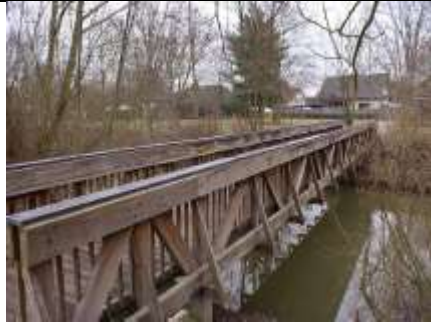
Fig. 5: Typical timber bridge to be inspected because of decay (although made by tropical hardwoods).
